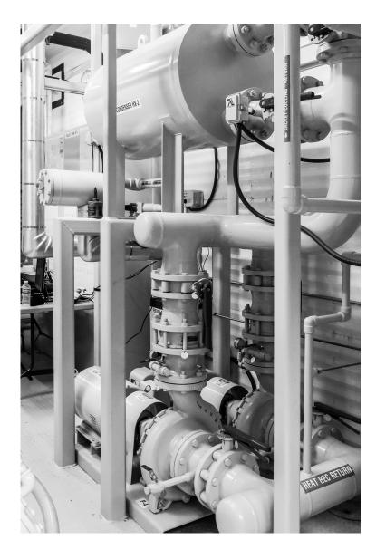
Accent Refrigeration's three most recent projects have been based on using Vahterus low-charge heat exchangers to improve safety and efficiency.
